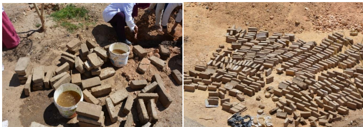
Figure- 7. Large-scale production of mudbricks based on the study's findings, with participation of students from the Conservation Department at Sohag University.
