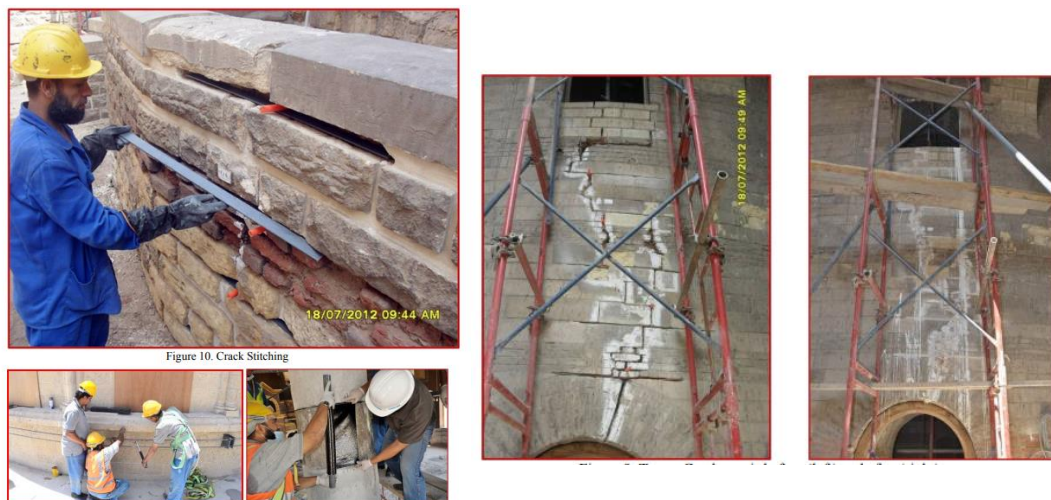
Fig (2,3): Restoration work on the Babylon Fortress tower
